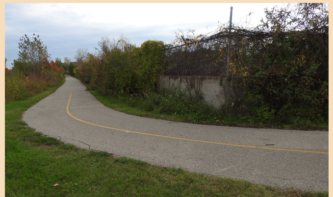
The concrete wall slated for removal.
