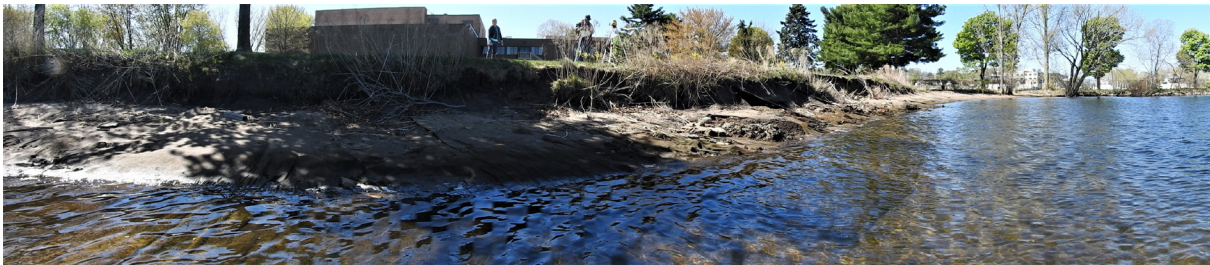
Pictured on left: Eroding shoreline at the Boys and Girls Club.
