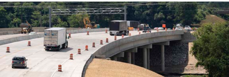
I-94 Grand River Bridge Construction, Jackson
