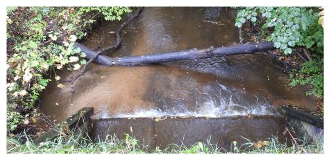
The box culvert at Roosevelt Road and Cushman Creek, a tributary of the White River, will be replaced with an open span timber bridge.
