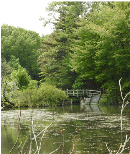
Ruckel's Bridge, Golden Township, Oceana County
