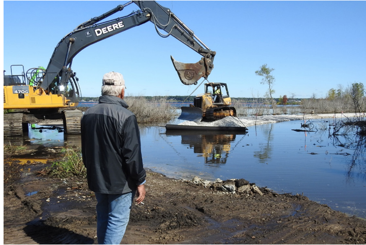
Greg overseeing construction efforts at the Amoco site.
