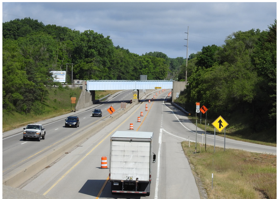
Road work on US 31 Business route
