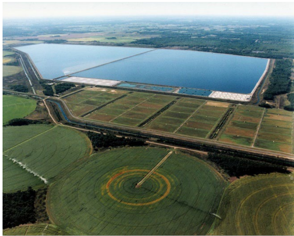
Muskegon County Wastewater Treatment Plant
