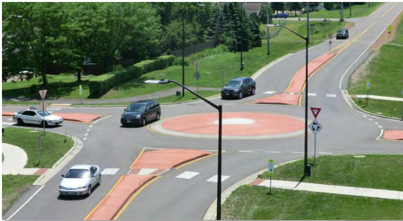
Figure 23 - Single Lane Roundabout (FHWA)
