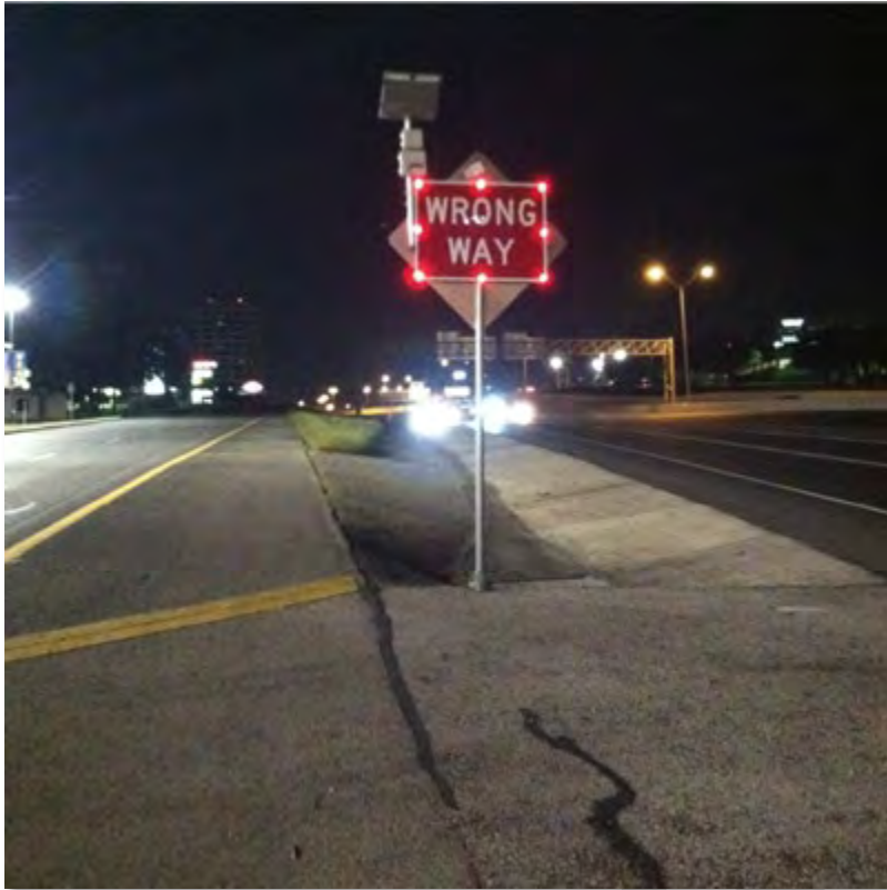
Figure 51 - LED Wrong Way Sign Installation (FHWA)
