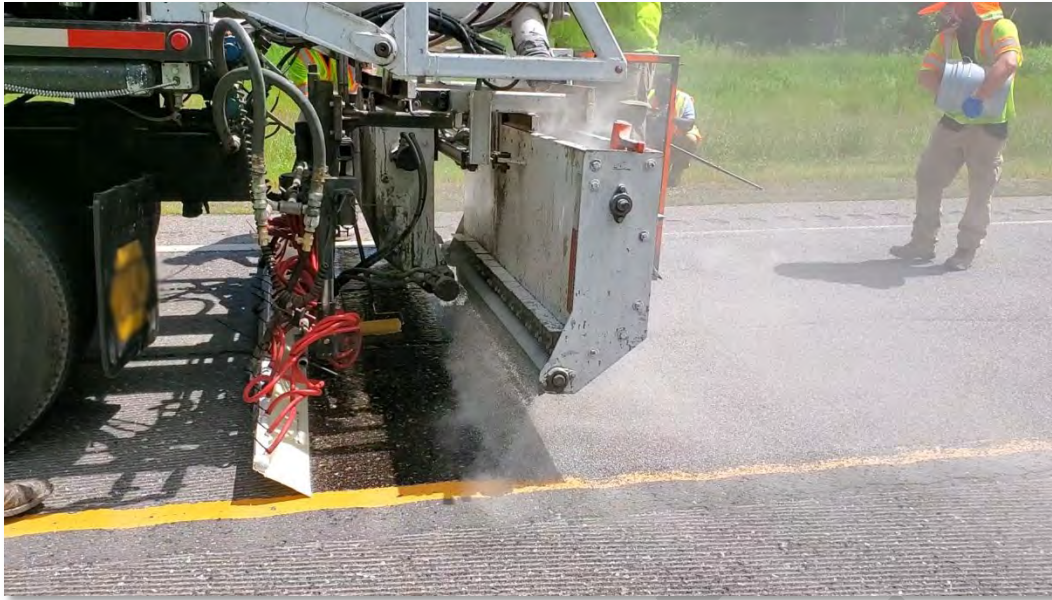
Figure 29 - High Friction Surface Treatment Application (FHWA)
