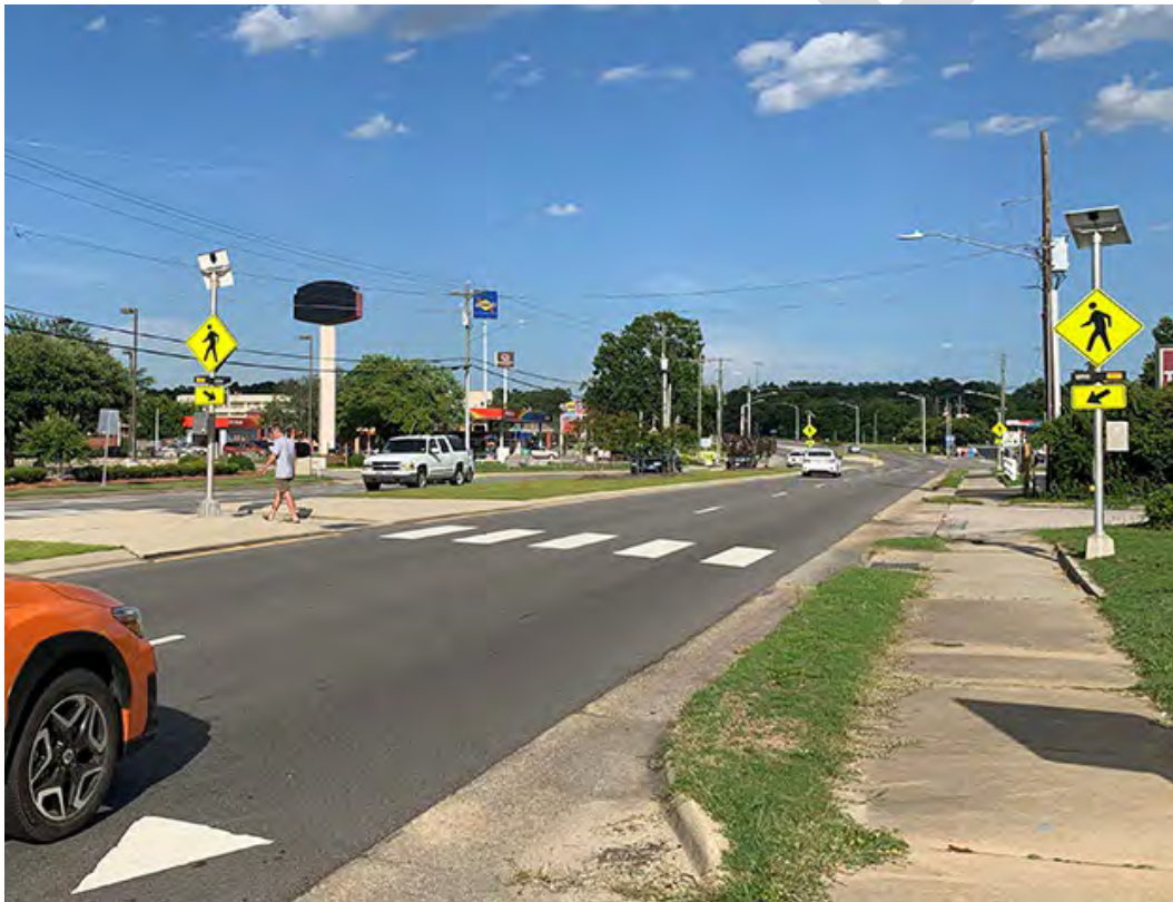
Figure 44 - Rectangular Rapid Flashing Beacon (RRFB) (FHWA)
