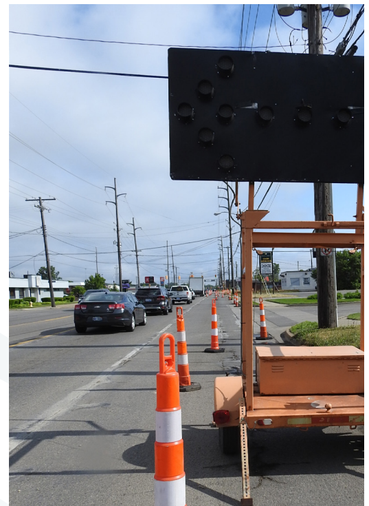
Preparation for roadwork on Henry Street in Muskegon
