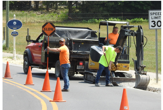
Roadwork in the City of Ferrysburg
