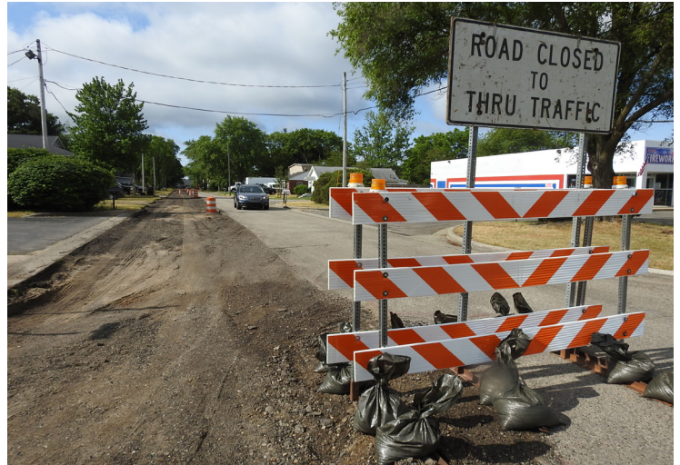
Road Construction in Muskegon County
