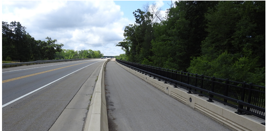
Stretch of highway US-231
