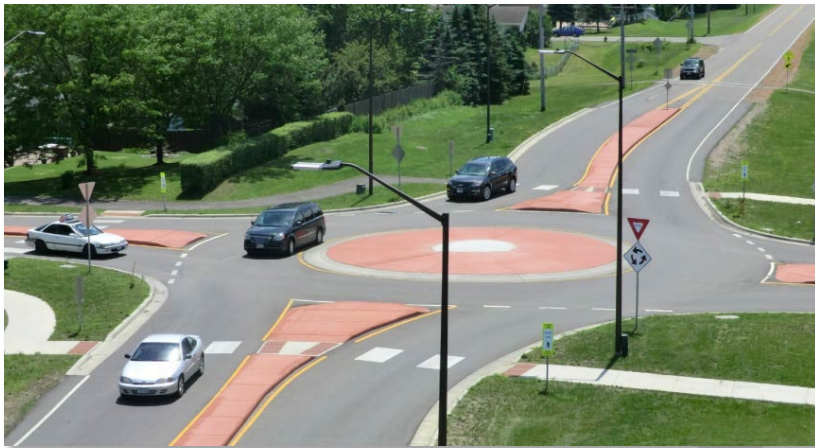
Figure 23 - Single Lane Roundabout (FHWA)
