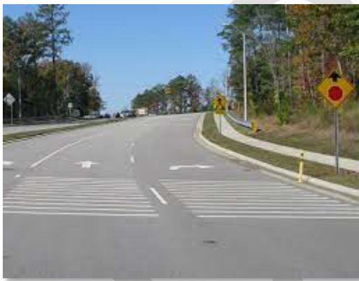
Figure 22 - Transverse Rumble Strips at Stop Controlled Intersection (ITE)
