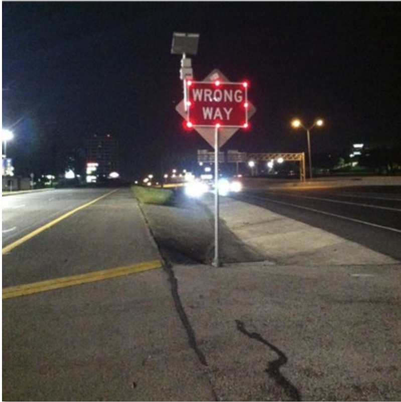
Figure 51 - LED Wrong Way Sign Installation (FHWA)
