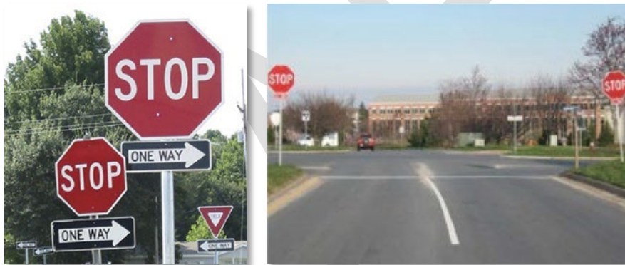
Figure 19 - Oversized Sign Comparison (Left, FHWA) & Double Stop Sign (Right, CFTR – Iowa State University)
