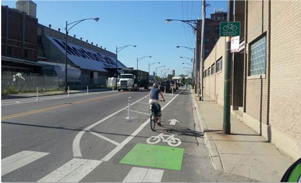
Figure 46 - Buffered Bike Lane (FHWA)
