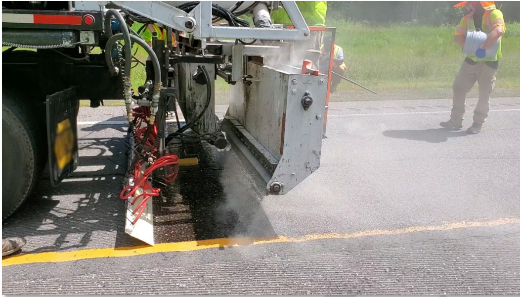
Figure 29 - High Friction Surface Treatment Application (FHWA)
