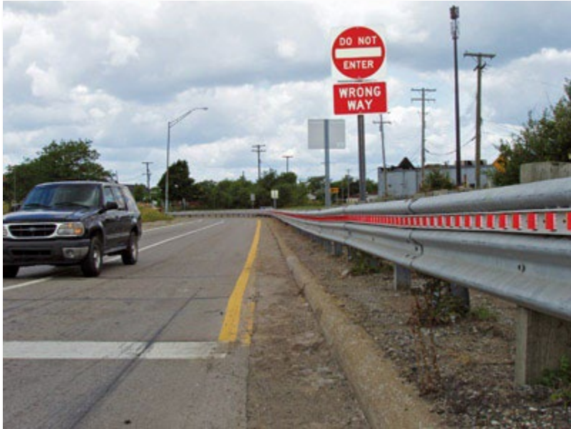
Figure 50 - Wrong Way Barrier Delineators (FHWA)
