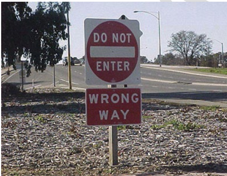
Figure 48 - Lower Mounting Height for Wrong Way Driving Signs (Caltrans)
