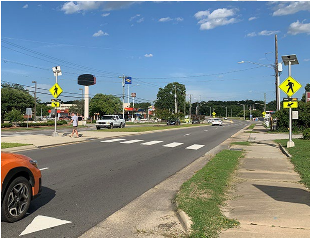
Figure 44 - Rectangular Rapid Flashing Beacon (RRFB) (FHWA)
