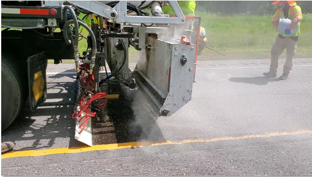
Figure 29 - High Friction Surface Treatment Application (FHWA)
