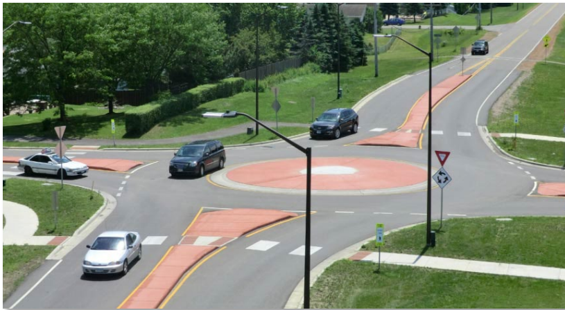
Figure 23 - Single Lane Roundabout (FHWA)
