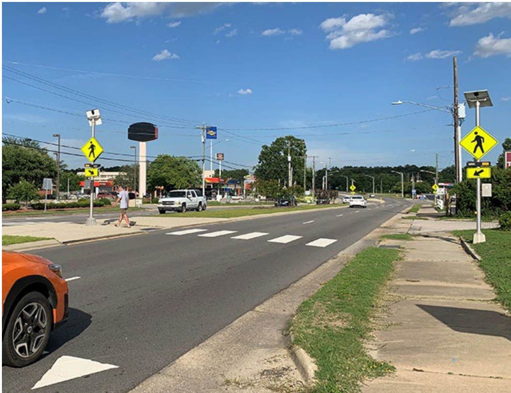
Figure 44 - Rectangular Rapid Flashing Beacon (RRFB) (FHWA)
