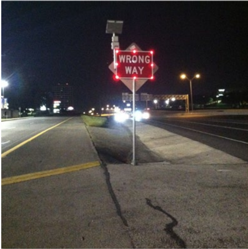
Figure 51 - LED Wrong Way Sign Installation (FHWA)
