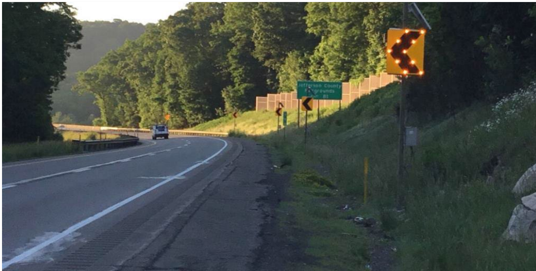
Figure 27 - LED Chevron Sign (PennDOT)
