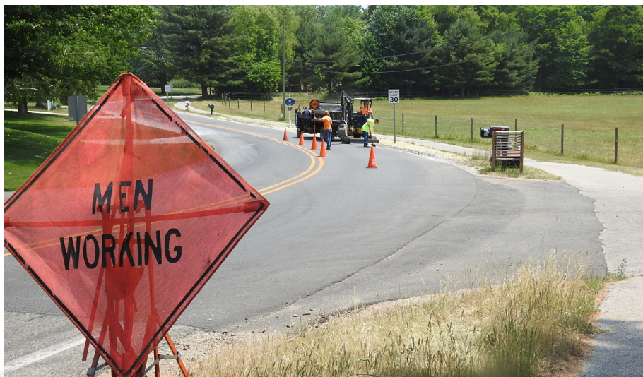
Road Construction in Northern Ottawa County
