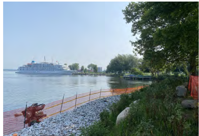
The shoreline conditions nearing the end of construction activities.
