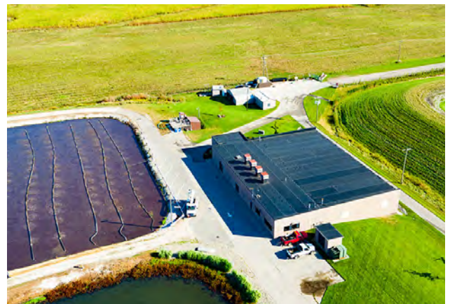
City of Hart BioPure wastewater treatment plant
