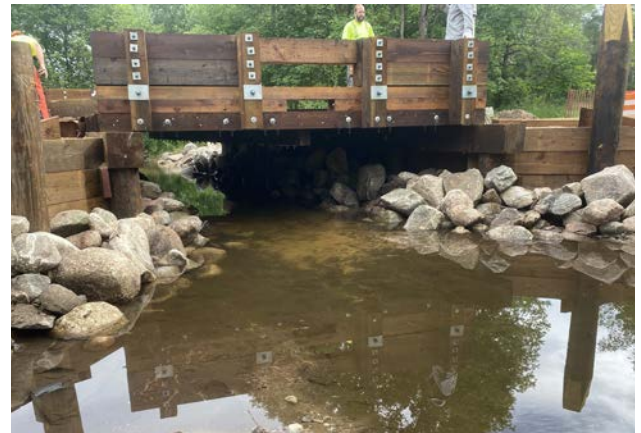
Open span timber bridge at Roosevelt Road and Cushman Creek
